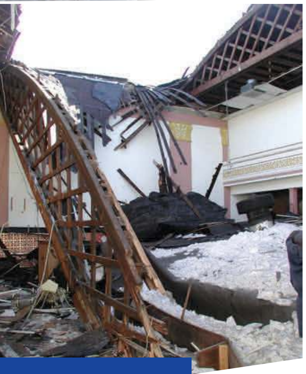
Top to bottom: A collapsed roof over an agricultural building that was the result of drifting snow in Minnesota; a church collapses as a result of excessive snow loads.
